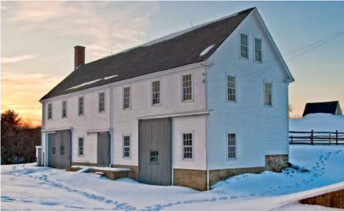
Squash House, constructed ca. 1915
